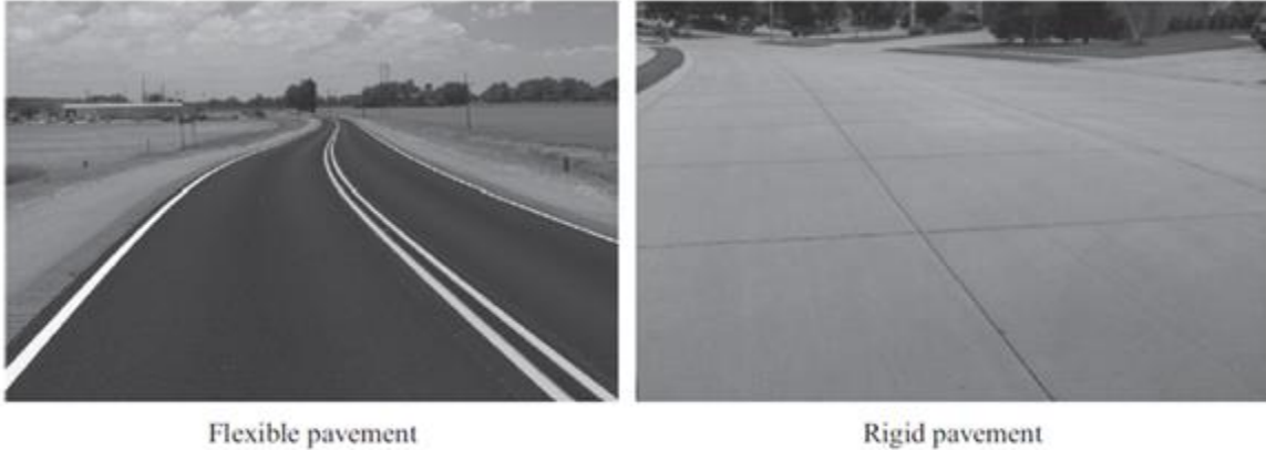
Figure 1 Flexible and Rigid Pavements
