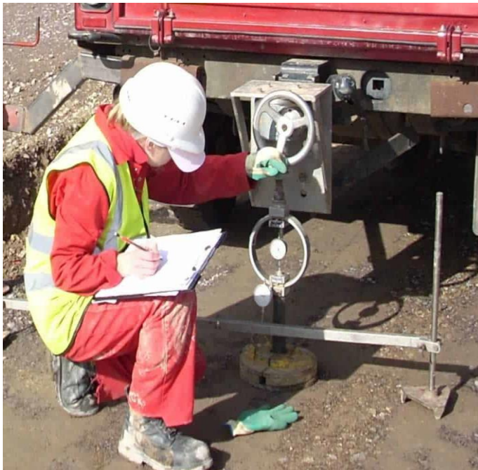
Figure 35 In Situ CBR Testing
